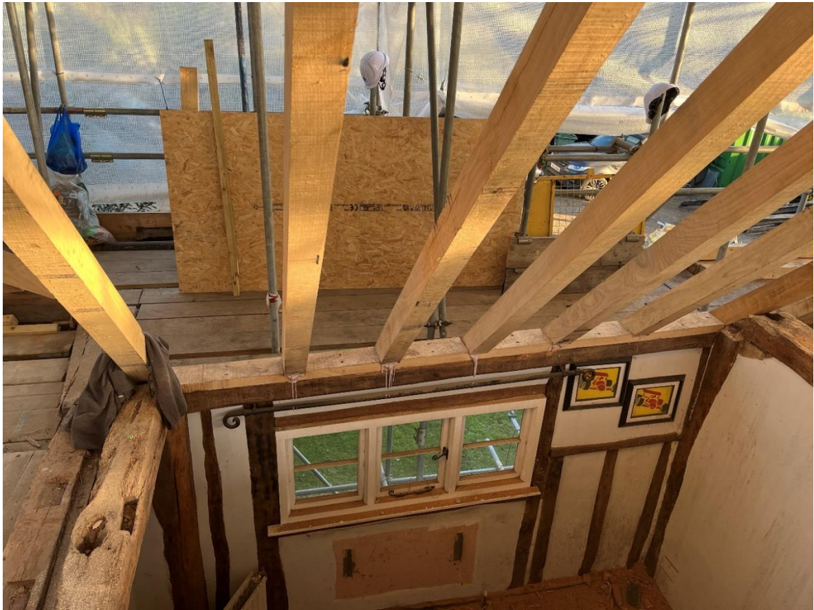
Site Photo 6. View across roof floor
