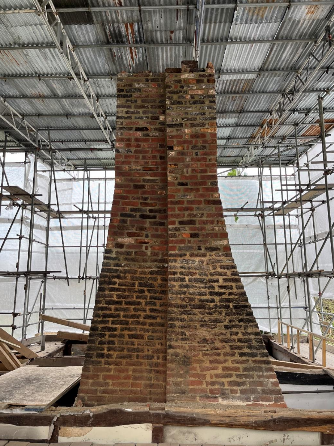
Site Photo 2. Northern Chimney Stack
