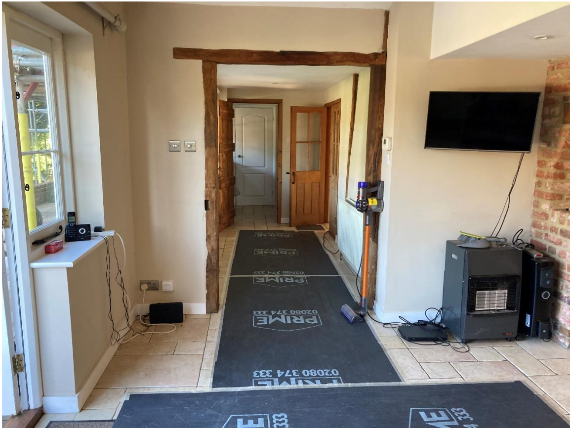
Site photo 12. Hall area (Looking NE)
