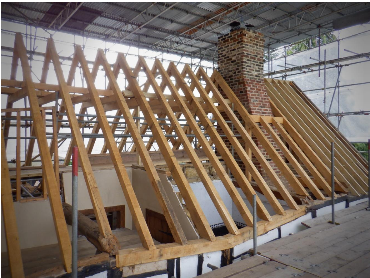
Site Photo 7. New roof on rear extension showing rear chimney
