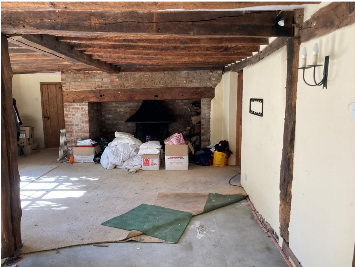
Site photo 9. Ground floor (looking SE)
