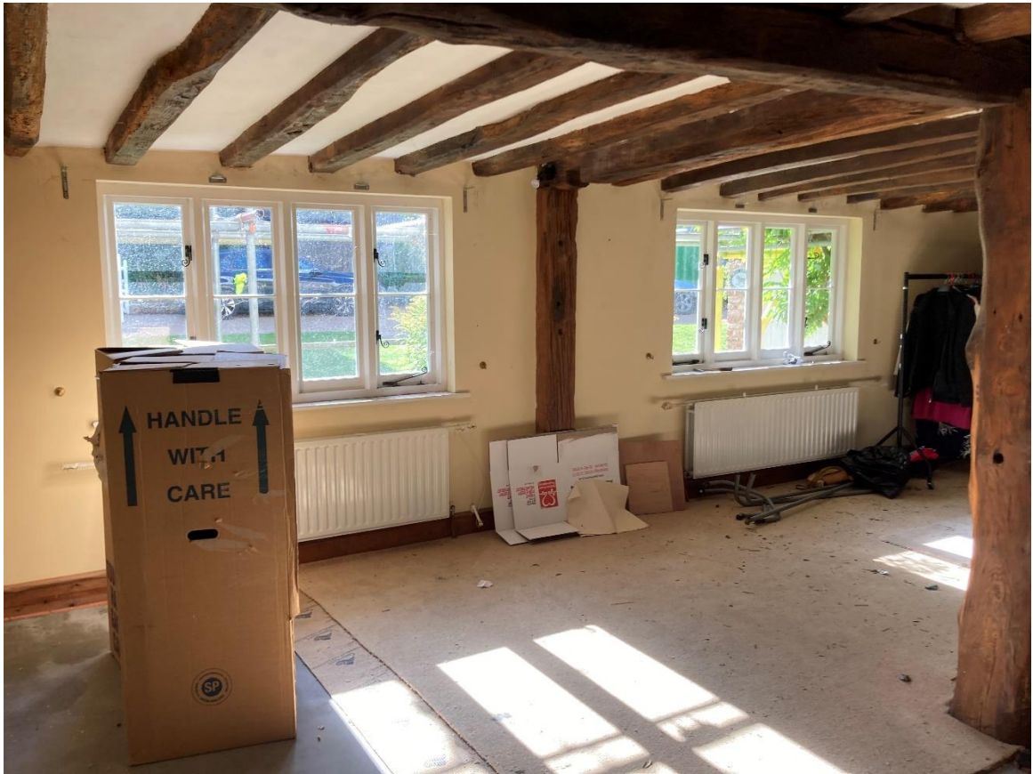
Site photo 10. Ground floor (looking west)
