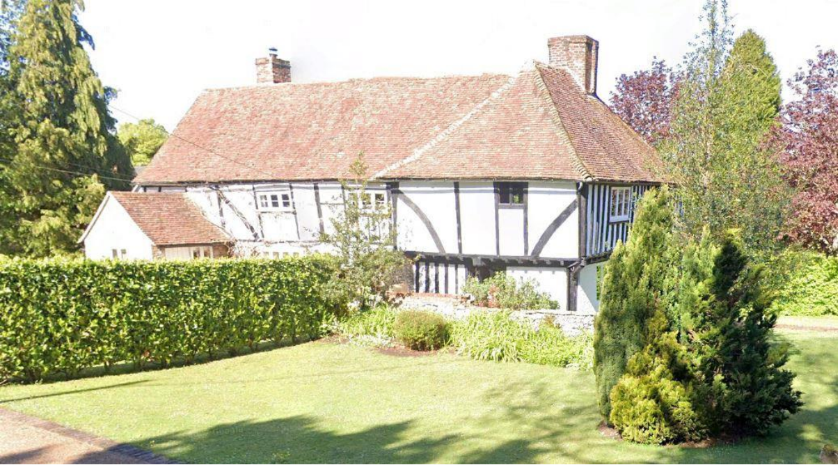
Historical Site Photo 2. Eastern Elevation May 2021
