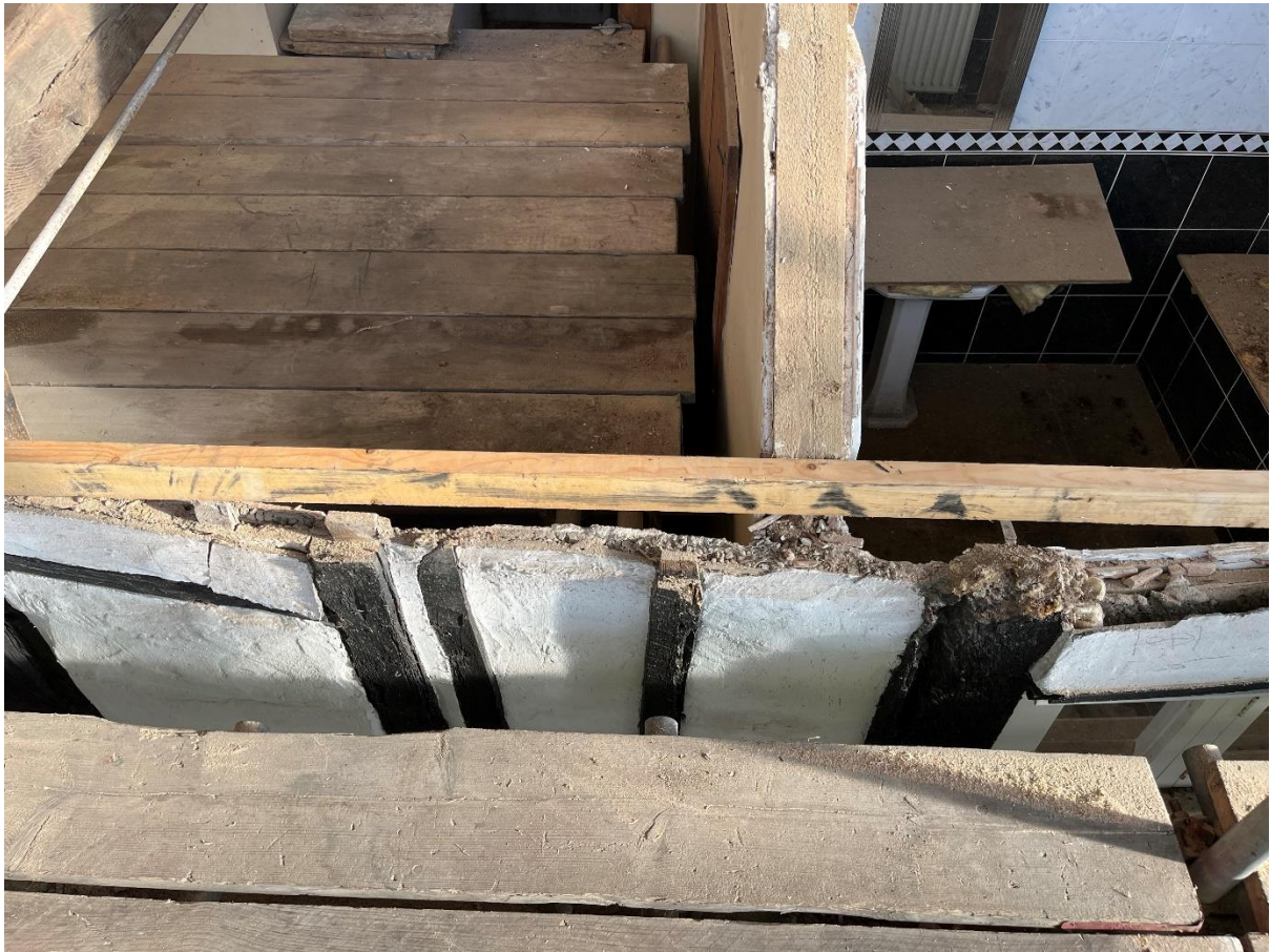
Site Photo 4. Detail of exposed building side.
