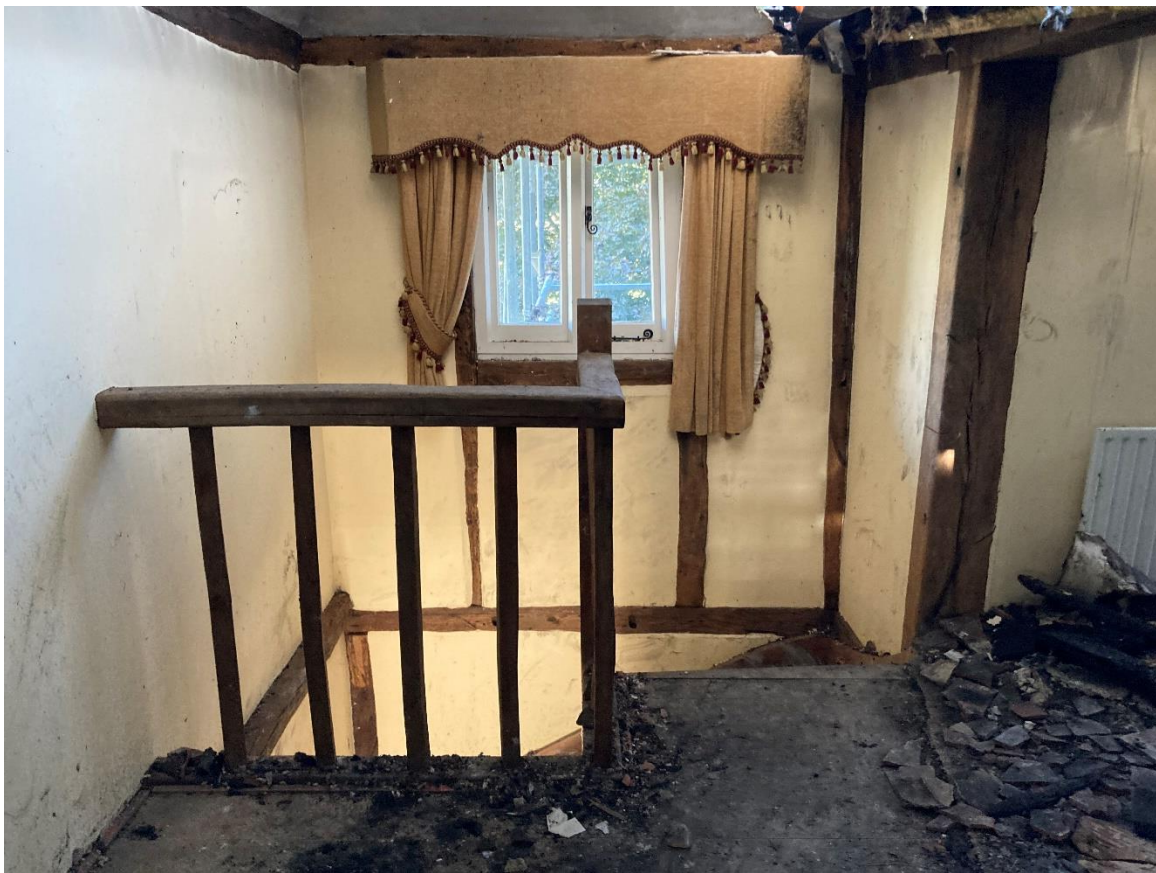
Site photo 13. Staircase area (Looking north)
