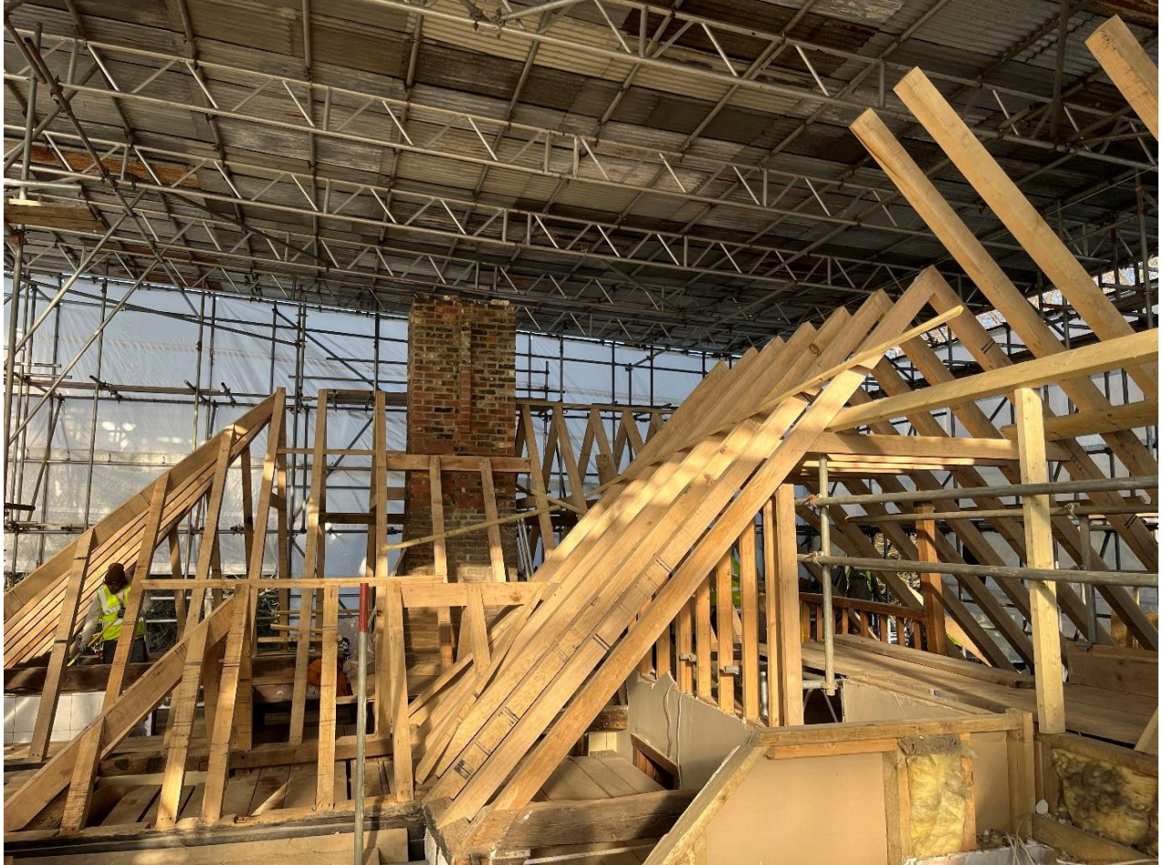
Site Photo 3. Rafters, Looking north
