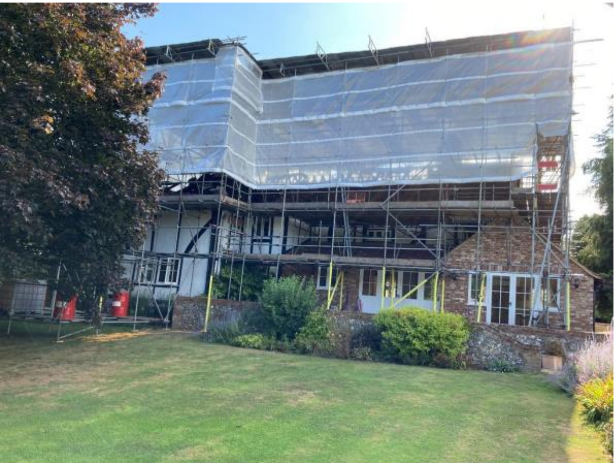
Site Photo 1. Western elevation
